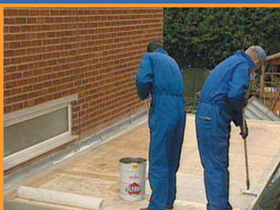
APPLYING THE NEW COMPOSITE
